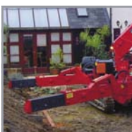
Level operation on uneven sites
